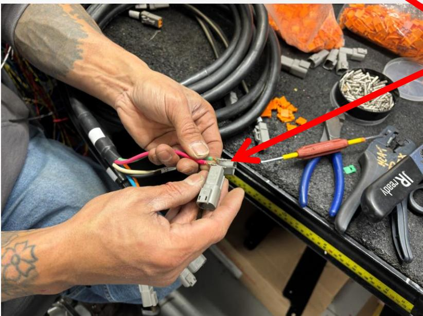
If the connectors on the end of the heat harness, do not match the heat element or heat box, complete the following process.
